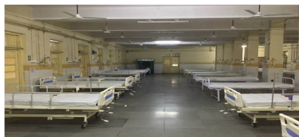
Figure3:plastic surgery wards were upgraded with central oxygen supply and suction system ports to each bed
